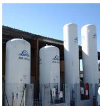
Monitoring and control of medical gas storage by collecting the data of temperature and pressure sensors. Our system allows to monitor the consumptions of gas and to avoid interruptions of delivery of gas for the hospital.
